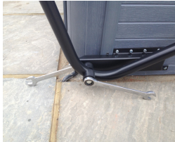
Install pivot arm using nut, blocks and washers
