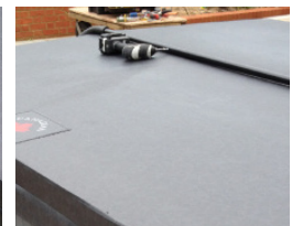
Screw in centre coupler - at a horizontal angle with screw heads facing the back of the spa
