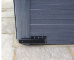
Mark drill holes & drill with # 8 drill & screw brackets to cabinet
