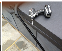
Screw in side arms using self tapping screws
