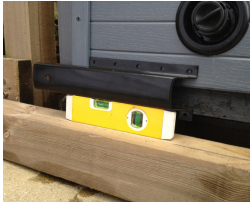
Ensure bracket is level on both sides
