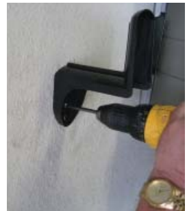
Fig. 4 Mount the hose hanger.
