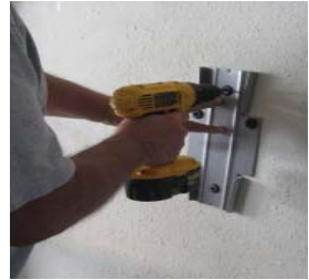
Fig. 2 Mount the wall bracket.
