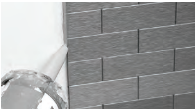
Finishing option 2: Caulking outside edges
