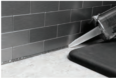
Caulking the countertop seam
