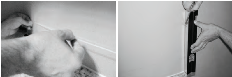
Mark horizontal and vertical reference points
