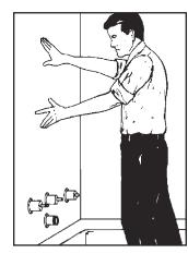
8. Trial fit each panel before proceeding. For an attractive installation, it is important that the top edges properly align.
