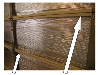
For improved thermal performance, add 3/4" air space between Reflective Air and door. This can be done by attaching to door framing rather than to the door panel
