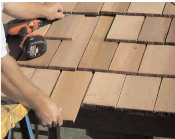
52. Roof Filler Shingles are included to cover roof seams. Starting at the bottom, slide the first Long Shingle in until flush with other bottom shingles. DO NOT ATTACH UNTIL STEP 53.
