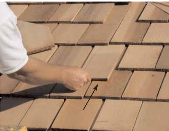
52. Roof Filler Shingles are included to cover roof seams. Starting at the bottom, slide the first Long Shingle in until flush with other bottom shingles. DO NOT ATTACH UNTIL STEP 53.
