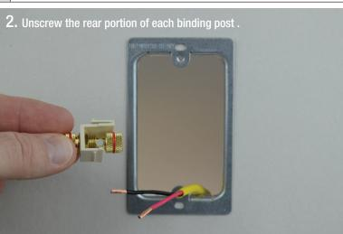
through opening on the side of the binding post.
