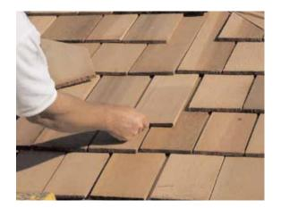
**41.** Slide in another Long Filler Shingle and attach as per **Step 40.** On your last row of shingles, the Filler Shingle is precut to fit properly. Attach to roof with 2 -1 1/4" finishing nails.
