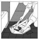
To make contoured and irregular cuts, use nippers to take small bites to prevent cracking or breaking of tile. With rod saw use long, even strokes to avoid binding. Smooth cut edges with an abrasive stone.
