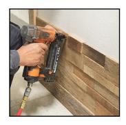
Hold the first panel in place at the bottom left of the first row to be secured.
