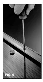
If the crown is raised also ensure the new height is not compromising proper door operation.
