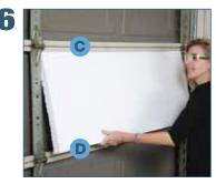
Insert the insulation sheet between horizontal rails C and D with the channeled or grooved side facing the garage door.
