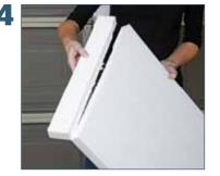
Break off the insulation where cut.
