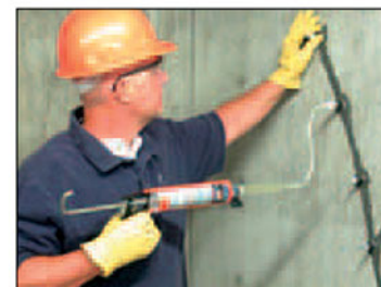
Crack-Pac® injection epoxy using the E-Z-Click Port System
