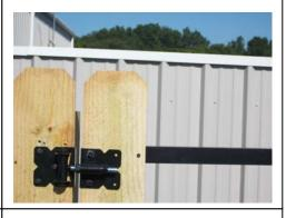
Step 12) Attach next board on the latch side of the frame.
