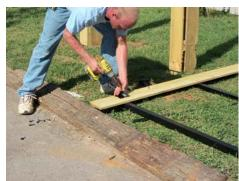
Step 11) Attach the gate brace diagonally to the vertical uprights on frame.
