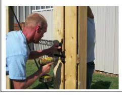
Step 8) Screw the hinges through the first board onto the Dura-Gate<sup>TM</sup> frame. (Be
