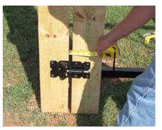
Step 13) Install the latch, striker bar, and handle to the post and gate at desired height. Then, install the remaining gate boards. \*
