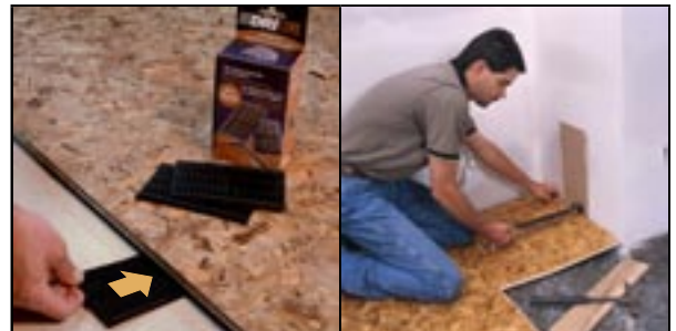
5. Use DRlcore shims for leveling
