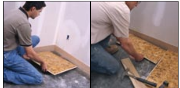
3. Install 1/4" spacers for expansion gap
