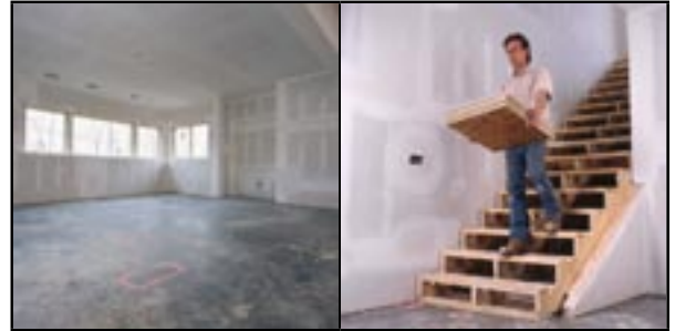
1. Clean floor. Level spots > than 1/4"
