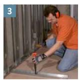
Attach floor runner using concrete anchors.
