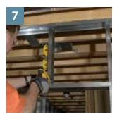
Cut and install runners and cripples around doors and windows.
