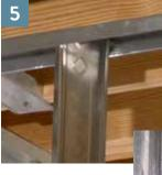
Twist studs into place. Make sure studs are level and knockouts/ punch-outs are aligned.
