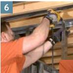
Screw studs to top and bottom runners using 7/16" pan screws.
