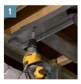
Attach ceiling runner to bottom of joist or truss.
