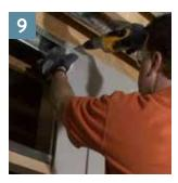
Attach drywall. Use corner bead around corners. Tape, spackle and finish drywall.
