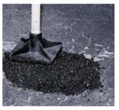
d. For holes larger & deeper than 1", use Ready Road Repair Pot Hole Patch. Use tamper to pack material tight into repair. Ready for traffic immediately. Allow to cure a minimum of thirty days prior to seal coating.
