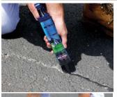
a. Fill cracks up to ½" wide with Black Jack Speed-Fill Crack Filler.
