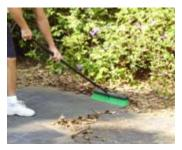
a. Sweep entire surface, removing grass cuttings and other debris. Scrape clean all cracks using a screwdriver.
