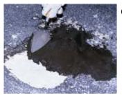
c. Repair large cracks, deteriorated surfaces,, and small holes up to 1" deep with Black Jack Speed Patch. Apply with trowel, tapering into existing surface.
