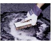
c. Scrub gasoline and oil stains with undiluted Driveway Kleen™ and a wire brush. Shoot stream of water into cracks and flush clean.
