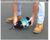
For expanding cracks or climates with wide ranges in seasonal temperatures, fill cracks up to ½" wide with Black Jack Speed-Fill Elastic Crack Filler.
