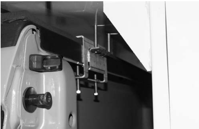
Figure 2-12 – Top Plate Bolts
