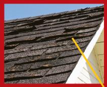
Missing, cracked or curling shingles. Possible cause: Shingles have reached their useful life.
