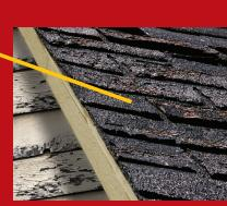
Roof shingle, sheathing and siding decay. Possible cause: Poor attic ventilation.
