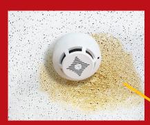
Stains on interior ceilings and walls or mold and mildew growth. Possible cause: Inadequate or faulty shingle underlayment allowing leakage, or inadequate ventilation.
