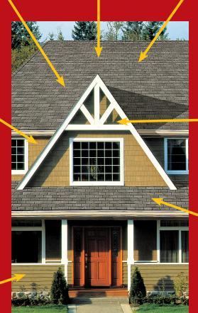
Leakage in attic after driving rain. Possible causes: Leaky or inadequate shingle underlayment; deteriorated flashing.
