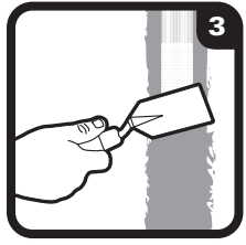
Fill gaps with FlexBond , embed mesh tape, smooth with trowel.
