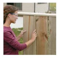
Install the posts, top and bottom rails, and a cap rail that overhangs the side of the rail on which you'll hang the fence boards. Cut the fence boards to length and tuck them under the cap rail, spacing them with the narrow edges of a batten. Plumb the boards with a level and fasten them with 15/8" deck screws.
