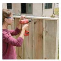
Cut the battens to length with a circular saw or power miter saw. Center each batten over the space between boards and screw it to the top rail. Plumb with a level, then screw to the lower rail.
