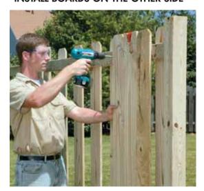
Go to the other side of the fence. Put the spacer against the first post, and install a board against the spacer. Install boards along the entire side, spacing them with the spacer.
