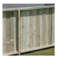
Like any other fence, this option is made of posts and rails. However, it's both more durable and more attractive thanks to a few changes; most importantly, the cap rail that runs across the top. The cap rail protects the tops of the posts, which absorb water more readily and are more likely to rot than any other surface of the post. The fence is also designed to look the same from both sides—your neighbor will likely appreciate that.
