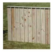
This fencing mimics the siding once applied to farm sheds, barns and similar outbuildings. The cap rail is an important part of this fence. Without it, each board's end grain would be exposed to the weather, and the life of the fence would be shortened.
