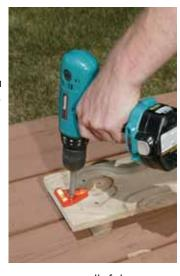
level to the spacer so you can tell if the boards are plumb before attaching.
