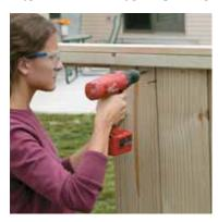
Put the first board in place next to a post, make sure it's plumb, and screw it to the supports with #8 1 5/8" deck screws. Work your way down the fence, using a nail as a spacer between boards (this allows them room to expand in humid weather. When you're done, screw a second set of 1x1 supports tightly against the fence boards.
