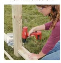
Install 4x4 posts and 2x4 top and bottom rails, then nail a 1x4 cap rail over the top rail. Cut two 1x1 supports to fit between each post. Screw the supports along the outside edge of the bottom rail on one side of the fence, fastening them every 6 to 8 inches with #8 2" deck screws. Repeat on the top rail.
