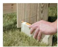
It's not always possible to remove rocks and other obstructions from the ground. If there's an obstruction you can't get rid of, cut the fence board to follow the shape of the obstruction. Lay out the cut by clamping the full-length board plumb and in position, then using a scrap 2x4 and pencil to scribe the shape of the ground onto the board. Make the cut with a saber saw, then trim the board to length and install it.
