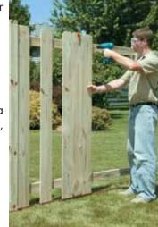
along the fence, positioning the spacer and screwing the boards in place.
