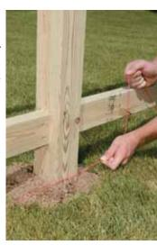
two below the top of the post to calculate the proper length of the fence boards.
