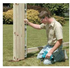
Align a fence board with the mason's line and butt it against the first post. Once you've made certain it's plumb, use #8 2" deck screws to screw it to the rails.
