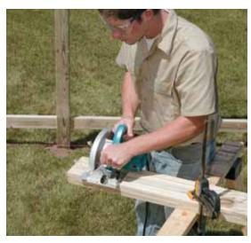
You can speed up the job by clamping two or three boards together and cutting them at the same time.
