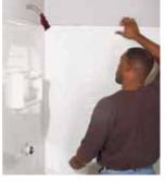
hand pressure over the surface, up and down and side to side, to ensure maximum contact. Remove excess adhesive. Do not use the shower for the next 24 hours. Install the fixtures after the adhesive has dried.
