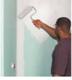
area, shut off the water supply and remove all fixtures. Clean the surface with denatured alcohol to ensure a good bond for the enclosure panels. Prime or water seal raw plaster, wallboard, or spackling before you install the panels.
