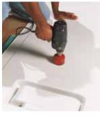
saw. Make the holes large enough to allow clearance for the pipe but small enough so the escutcheon completely covers the hole. To avoid chipping the surface while drilling, drill from the back side of the panel. Test-fit the panel against the wall and check for accuracy by lining up the edge with the marked vertical line.
