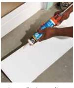
and press it firmly onto the wall, then pull it back about 6 inches for a few minutes (or per the manufacturer's instructions) to let the adhesive set up. This will provide a permanent bond. Push the panel back in place and apply pressure with your hands, up and down and side to side, making sure that all areas of the panel are in firm contact with the wall.
