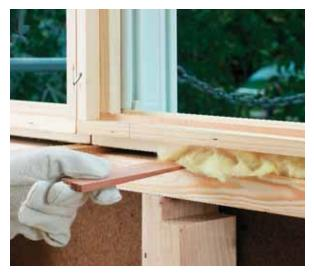
**FILL THE GAPS BETWEEN THE WINDOW JAMBS** and the framing members with loosely packed fiberglass insulation. Wear work gloves, safety glasses, and a dust mask when handling insulation.
