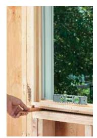
uneven, correct it by shimming below the side jambs and then tacking in place. Wear ear and eye protection when working with power tools.
