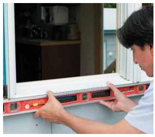
CHECK TO SEE HOW MUCH ADJUSTMENT WILL BE NECESSARY to level and plumb the window unit.
