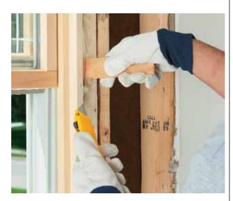
**TRIM THE SHIMS FLUSH WITH THE FRAMING** by scoring them with a utility knife and then snapping off the excess.
