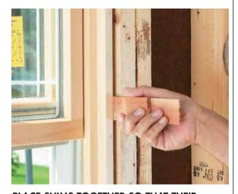
PLACE SHIMS TOGETHER SO THAT THEIR COMBINED THICKNESS WILL FILL THE OPENING BETWEEN THE JAMBS AND FRAMING. Despite the nails you just put in, the window will still move somewhat. Use the shims to center the window in the opening.
