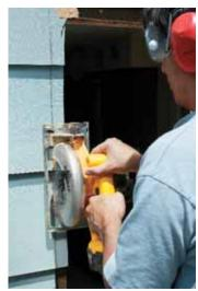
plate above the surface. Slide the saw guard back, start the saw, and ease the blade into the wood. To avoid splintering, stop before the corner. Complete the corner cuts with a sharp chisel.
