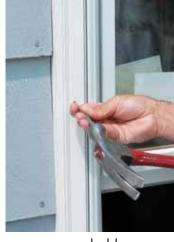
the remaining nails as recommended by the manufacturer. Drive all nailheads below the wood surface with a nail set.
