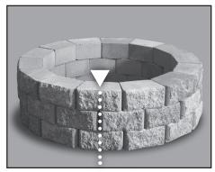
**7.** After the 2nd layer is finished, install the 3rd by placing the center of each block in line with the joint of the blocks below. When the 3rd course is all lined up, glue the blocks one-at-a-time as in step 6.
