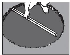
2. Check the level of the soil inside the circle in all directions. Remove soil from the high spots to bring it close to level.
