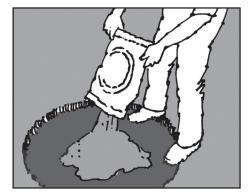
3. Add 1.5-2 inches of paver base to your circle and rake it level. Using a tamper, pack the entire area of paver base until firm. Make sure the surface is level before laying blocks.
