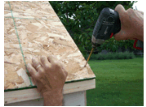
Step 13: Install large OSB roof section and fasten to rafters along bottom as shown.
