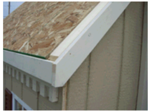
Step 24: Align gable trim as shown and fasten to building using 1-1/2" trim nails.
