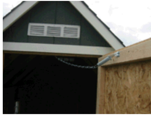
Step 32: Install door stop as shown, centering brackets on door and door header. Note: Keep bracket on door down at least 1-1/2" to prevent bracket from hitting door header.
