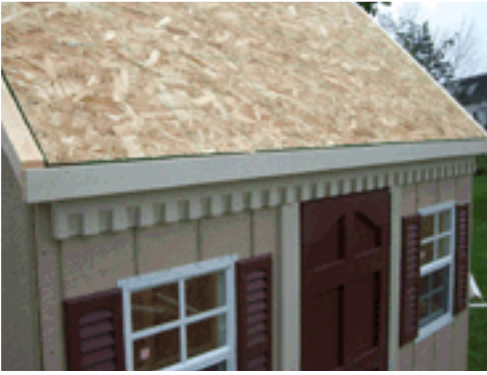
Step 23: Front fascia trim complete, repeat steps on back wall.
