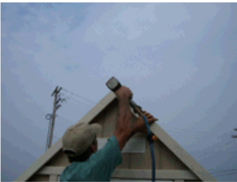
Step 26: Aligns back gable trim piece and fasten to building using 1-1/2" trim nails as shown. Repeat on opposite gable end.
