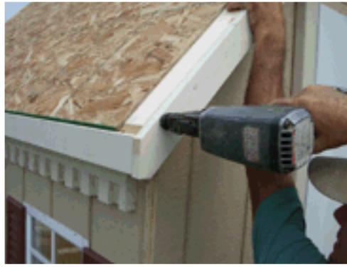
Step 24: Align gable trim as shown and fasten to building using 1-1/2" trim nails.
