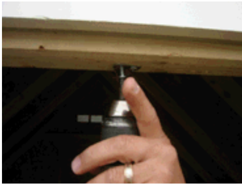
Step 30: Install door handle for large door as shown. Note: When installing inside of door handle, keep interior and exterior handles vertically aligned as shown.
