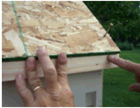
Step 13: Install large OSB roof section and fasten to rafters along bottom as shown.
