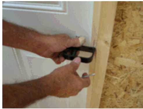
Step 30: Install door handle for large door as shown. Note: When installing inside of door handle, keep interior and exterior handles vertically aligned as shown.
