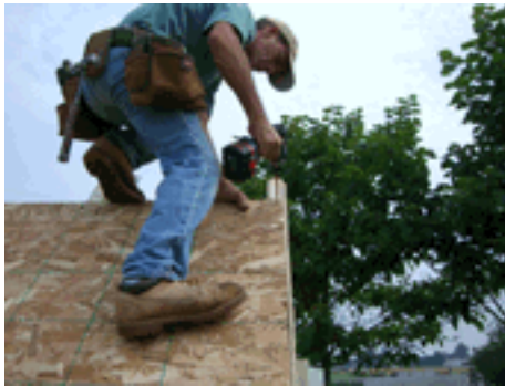
Step 14: Fasten edge of OSB to end rafter as shown.
