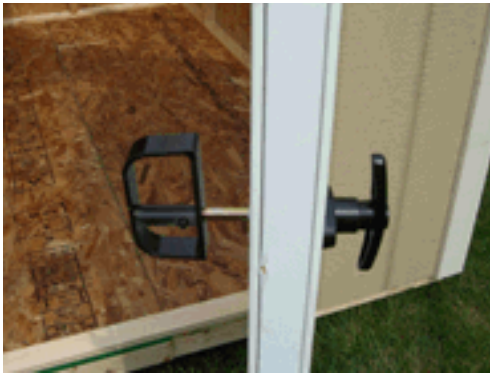
Step 30: Install door handle for large door as shown. Note: When installing inside of door handle, keep interior and exterior handles vertically aligned as shown.
