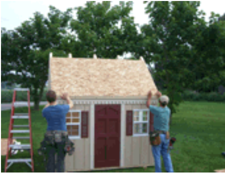
Step 13: Install large OSB roof section and fasten to rafters along bottom as shown.
