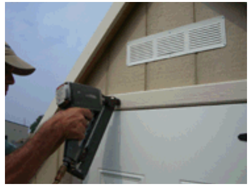
Step 25: Install top door trim before installing back gable trim and fasten to building using 1-1/2" trim nails.
