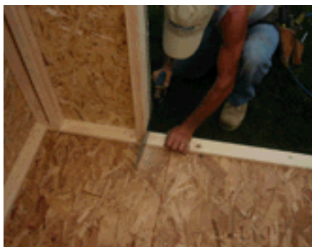
Optional door kick removal: It is recommended to remove door kick from side and front doors (this should be completed after roof is set).
