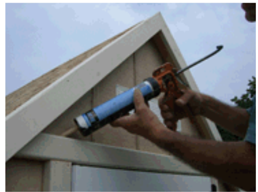
Step 27: Caulk above top door trim piece using clear silicone sealer as shown.
