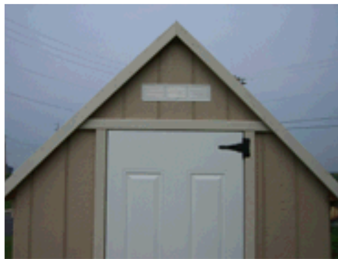
Step 26: Aligns back gable trim piece and fasten to building using 1-1/2" trim nails as shown. Repeat on opposite gable end.
