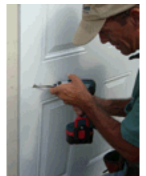
Step 18: Remove screw from door as shown.
