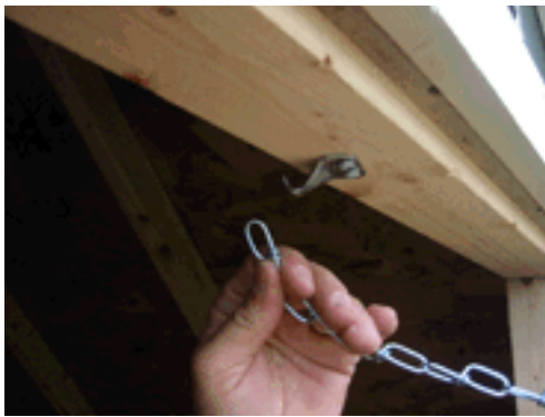
Step 32: Install door stop as shown, centering brackets on door and door header. Note: Keep bracket on door down at least 1-1/2" to prevent bracket from hitting door header.
