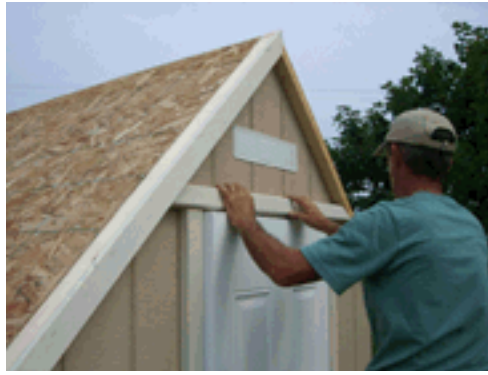
Step 25: Install top door trim before installing back gable trim and fasten to building using 1-1/2" trim nails.
