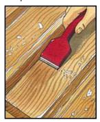
Any stubborn flecks that remain can usually be removed by using just the scraper. Again, be careful not to damage the work surface. When the paint is all gone, wash the surface with denatured alcohol or mineral spirits.
