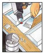
Hold the putty knife at about a 30-degree angle and, use it like a plow to push the paint away. Avoid gouging the wood. Dump the softened paint sludge into an old coffee can as you work. Special paint scrapers with angled blades work better than most ordinary scrapers.
