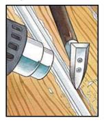
You'll want to go back over detailed areas with the heat gun, using a contoured scraper to get into narrow crevices.
