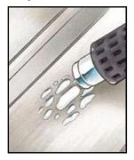
With the heat gun running, point the nozzle at the work surface, keeping it about 2 inches away. Move the gun back and forth across the surface until the paint begins to bubble and blister. Stop if the finish begins to smoke!
