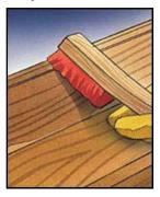
Scrub the entire project with nylon brushes or abrasive pads to remove all traces of the old finish and the stripper sludge.
