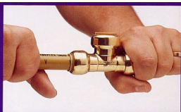
Push the tube firmly with a twisting action until it reaches the next Safe Seal Indicator Mark.
