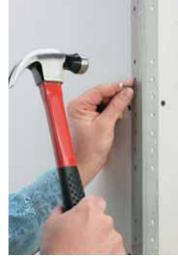
ceiling. Screws will distort the bead, so nail it in place, spacing the nails every 9 inches.
