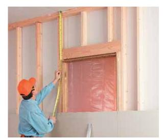
IF THE WINDOW IS ALREADY IN PLACE, TAKE OFF THE WINDOW TRIM AND CUT THE DRYWALL BEFORE YOU HANG IT. Lay out the cut by positioning the sheet along the floor and marking where it meets the edge of the windows. Measure from the ceiling to the window top to lay out the top of the cut.
