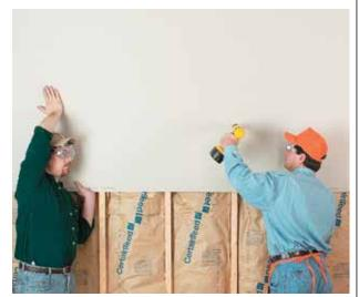
**MEASURE THE WALL** and cut the sheet so it's about 1/4 inch shorter than the opening. Have someone assist you in placing the sheet tight against the ceiling, and begin driving 1 1/4-inch screws in the middle of the panel.
