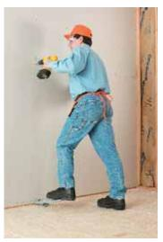
leave about a 1/2-inch gap. Position the lower sheet of drywall by slipping a panel lifter under the bottom edge and stepping on the lifter, then screw the panel in place.
